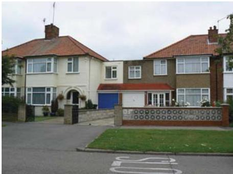
**Figure 38** This is an acceptable first floor side extension where the gap between the two dwellings has been retained by setting the extension in from the shared boundary
