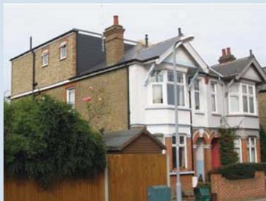
**Figure 45** A mansard roof extension which is at odds with the existing roof form
