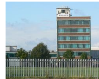
Towards the industrial estate
