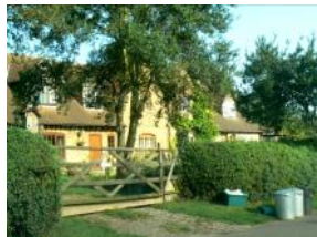
Tolworth Court Farm
