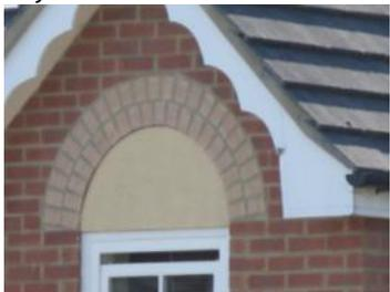
Thoughtless detailing—what purpose a lintel supported arch or a blind lancet window?
