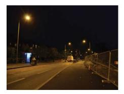
Road and new cycle path illuminated using 10m street lighting columns.
