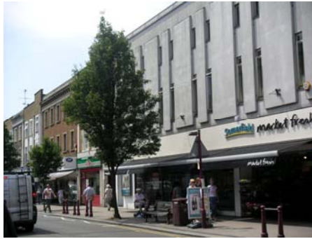
Somersetfield (Nos 15-17 Victoria Road)
