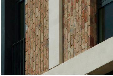
Figure 4.135: Stone / precast concrete coursings.
