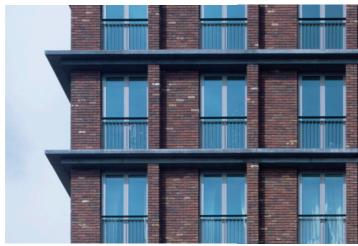
Figure 4.136: Stone / precast concrete coursings.
