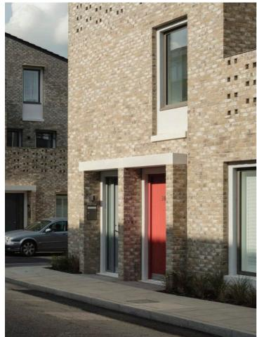
Figure 4.133: Stone / precast concrete features (lintels & sills).
