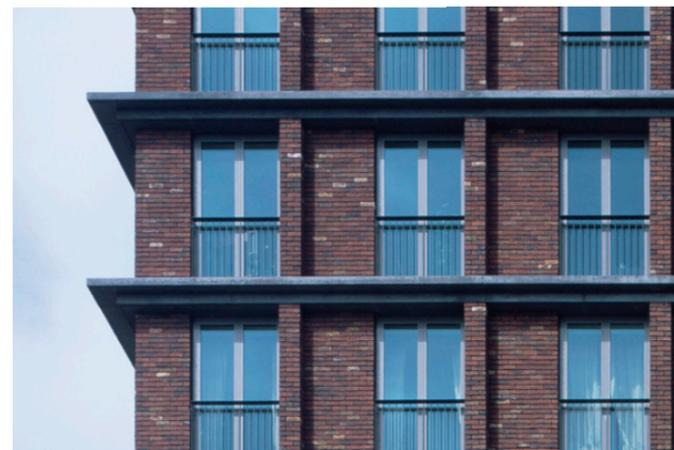
Figure 4.136: Stone / precast concrete coursings.
