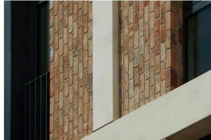
Figure 4.135: Stone / precast concrete coursings.
