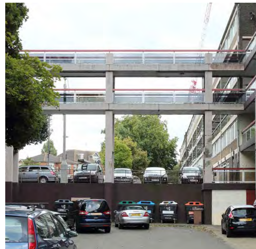
Figure 7.75: Existing elevated corridors
