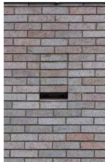
Figure 7.66: Integrated facade bat boxes
