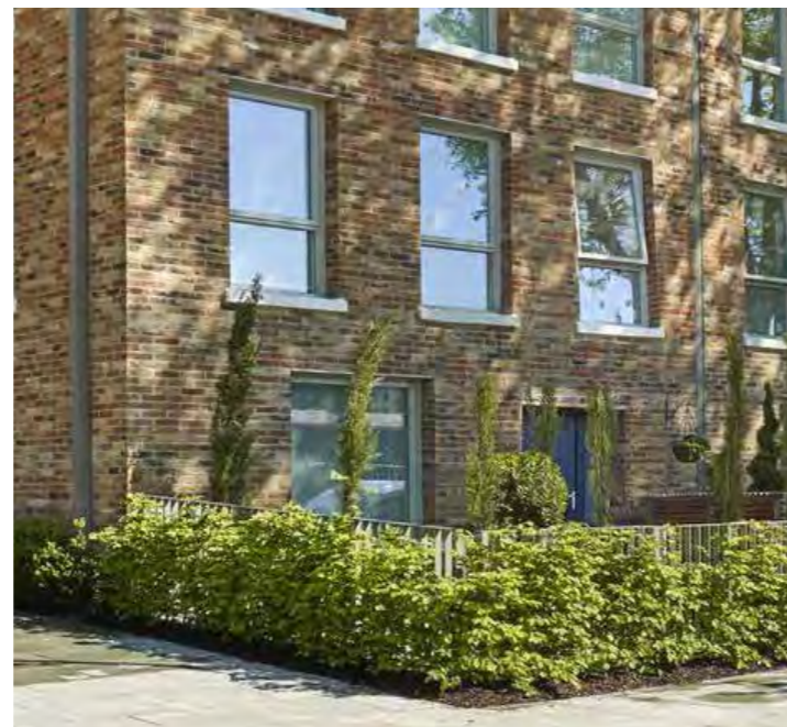
Figure 7.13: Type A precedent: metal railings with planting on the outside.
