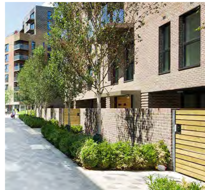
Figure 7.14: Type B precedent: brick wall and planting
