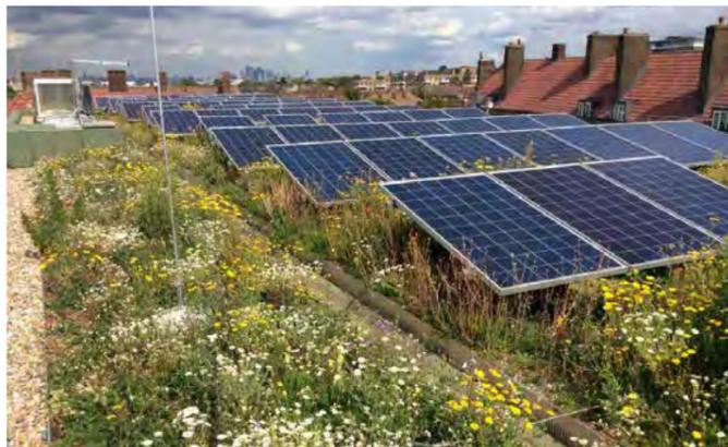
Figure 5.14: Biosolar roof. Photovoltaic panels and biodiverse roof.
