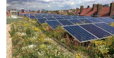
Figure 5.14: Biosolar roof. Photovoltaic panels and biodiverse roof.
