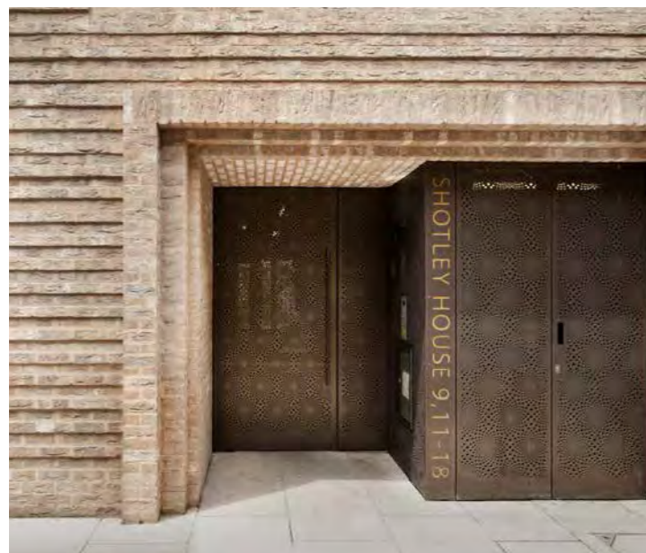
Figure 9: Recessed and expressed common building entrances .
