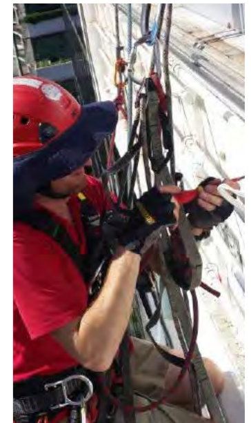
Figure 52: Facade access by abseil.
