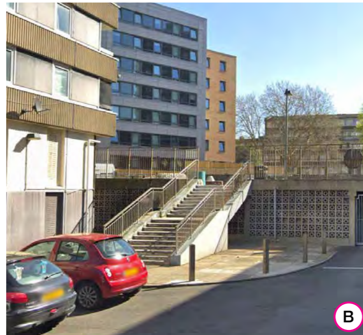
Figure 3: Existing level change.
