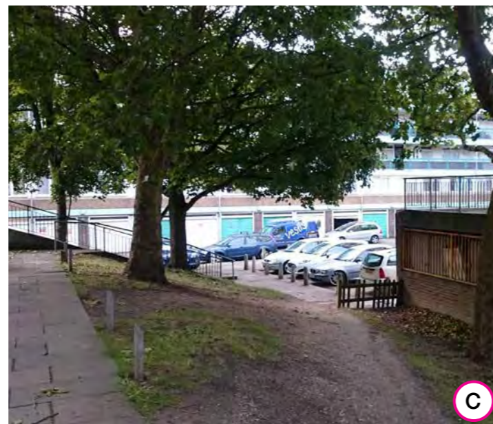
Figure 4: Existing level change.
