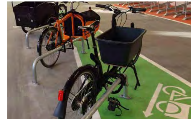
Figure 22: Staple parking hoops for transport / accessible cycles.
