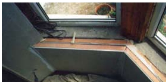
Figure 3.7 Insulation around window bay
