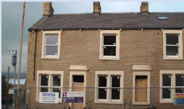
Refurbishment nearing completion
