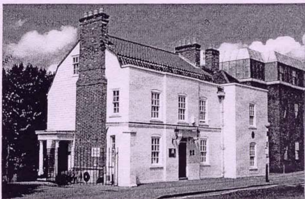
Picton House in the High Street, Kingston, as it is today.
