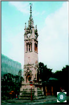
Surbiton Clock Tower., Claremont Road.
