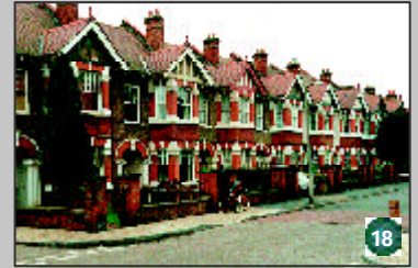
Lime Grove, The Groves.
