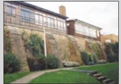
Listed wall near Kenry House, Kingston University.
